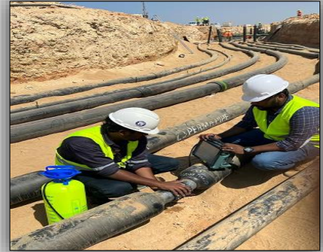
NDT Crew performing Phase Array Ultrasonic Test (PAUT)
